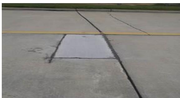
Gambar 6. Tambalan (*Patching end Utiliti Cut Patching*)
