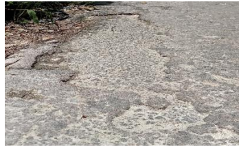
Gambar 6. Disintegration
